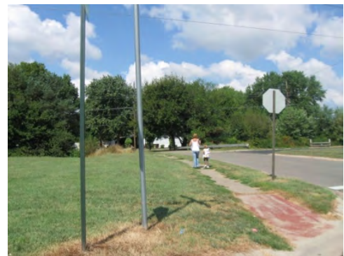
The sidewalk located on Eastgate Drive at Lockerbie Drive is inadequate.
